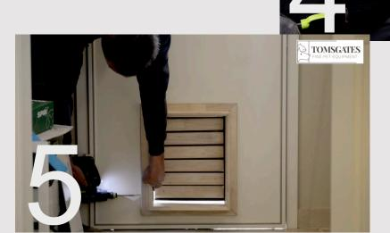
slide up and tighten the inner frame
